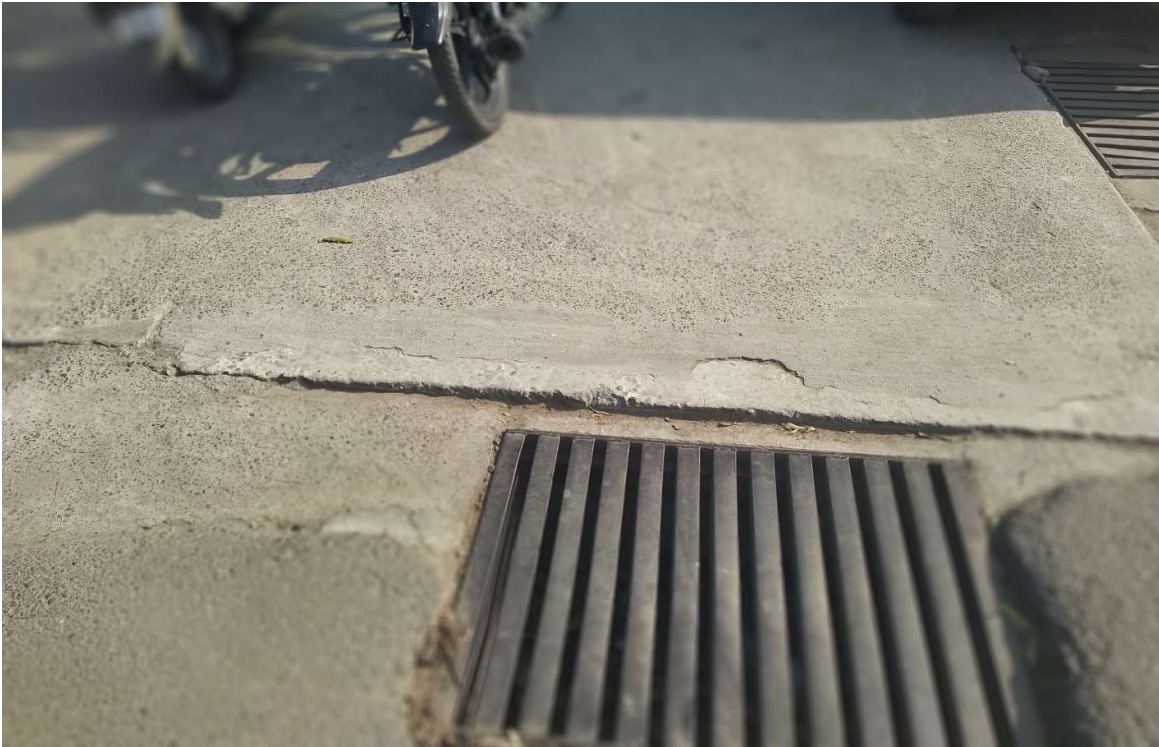
Rain Water Harvesting Systems at Khalsa college
